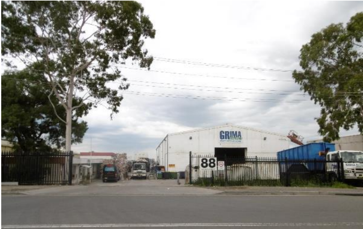
Figure 2.5. Entry to the site. Office and mechanical workshop are positioned on the left-hand side, and the paper and cardboard drop off, sorting and bailing warehouse is on the right.
